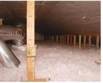
Making the improvements. Sealing leaky windows and air ducts, and adding insulation are the most common improvements auditors suggest. Attics can be the largest culprit for air and energy loss. For more on sealing and insulating an attic, see "Attic-Insulation Upgrade" on pp. 68-73.
